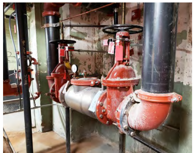
Fire Service Backflow Preventer
