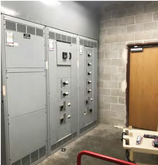
Main Switchgear
